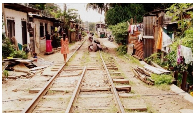
Photo 3: Current condition of the railway from Maradana to Homagama section
